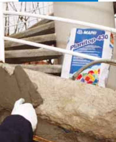
Application of Planitop 430
