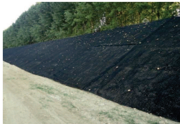
Installation of X-Grid AM
