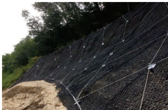
Installation of K-Mat RF Metal
